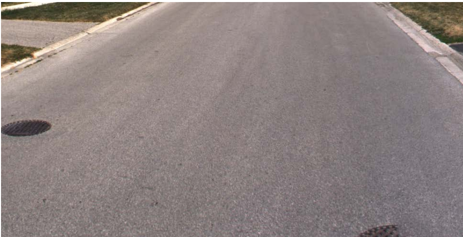
Brett Street - Very Good Road Condition
