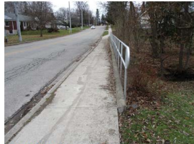
South Retaining Wall at West End
